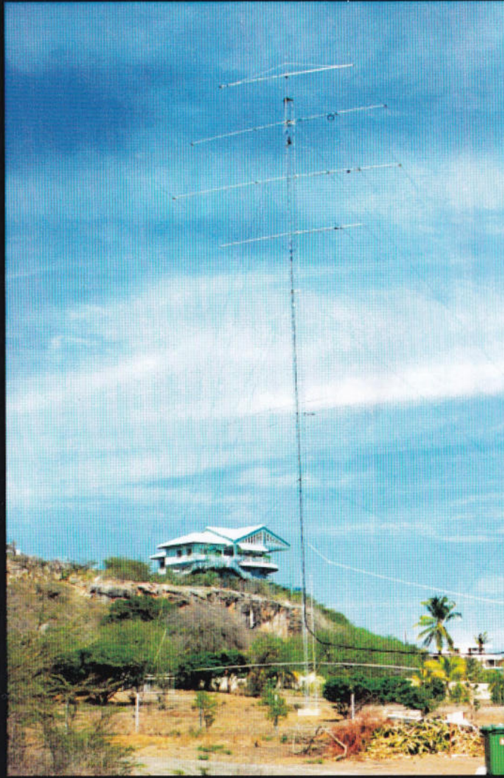
Views of the Main 100ft Tower - 5 element monoband beams for 20m, 15m, and 10m fixed on Europe plus A3S for South America
